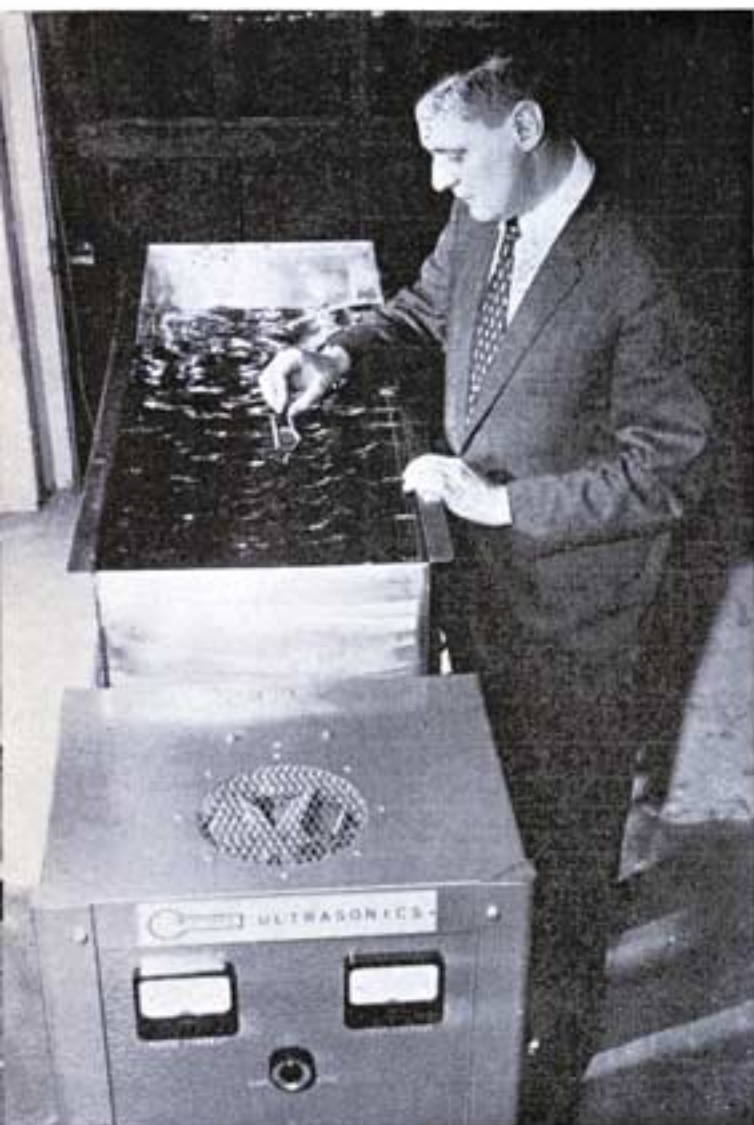
Hundreds of camera lenses which are caked with hard pitch used to hold them during grinding, are dipped into this ultrasonics tank for a final cleaning operation.
